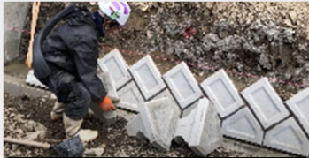
Installation and removal of stone, etc.
