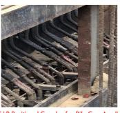
WK.LP Positional Coupler for Pile Cap Application (When both rebars cannot be rotated)
