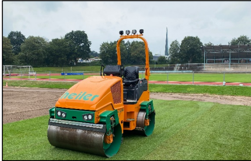
Landscaping and turf construction
