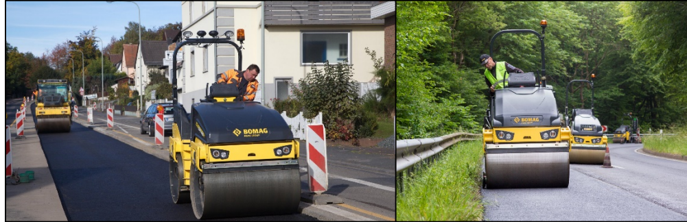
New road construction and repair
