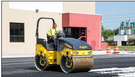
Carpark & industrial yard construction
