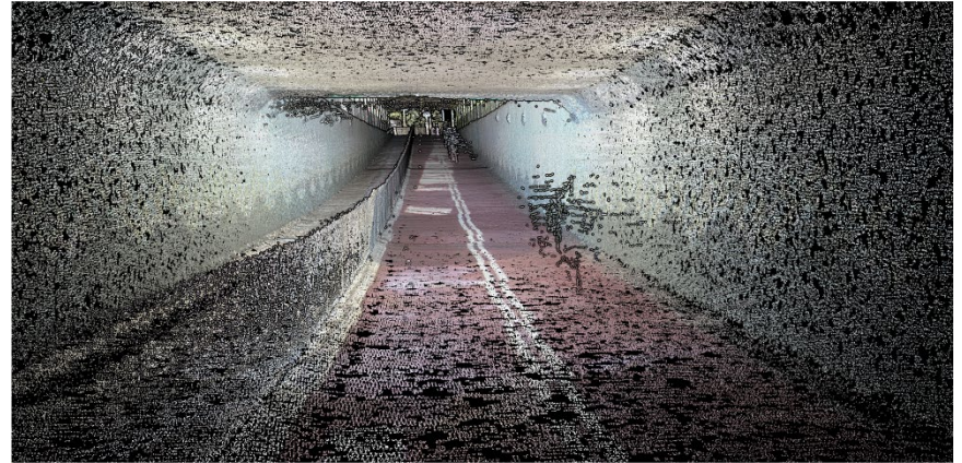
Point Cloud of pedestrian and bicycle tunnel near Sheung Shui
